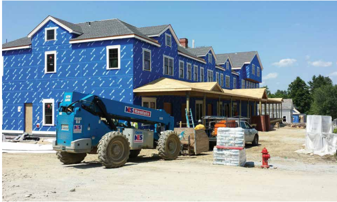
During construction of the new hotel, it wore a blue skin to self-adhere to a substrate and provide a waterproofing barrier.
